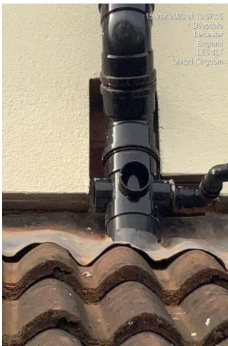
Figure 10 a), b) & c) Various locations of soil vent pipes junctions resulting in thermal bridges
