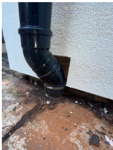
Figure 10 a), b) & c) Various locations of soil vent pipes junctions resulting in thermal bridges
