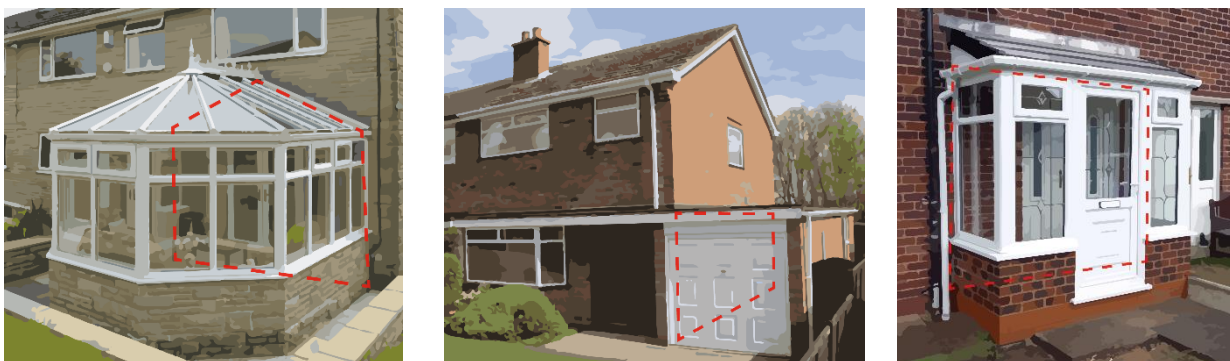
Figure 8 Examples showing the internal heat loss walls in the red dotted area requiring insulating
